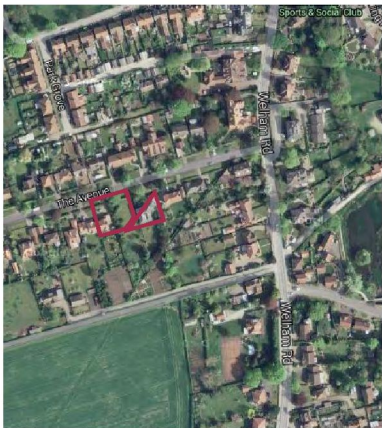
Aerial view noting site
