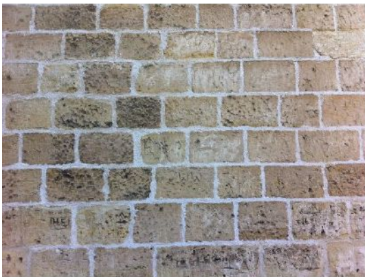
Lime mortar pointing
