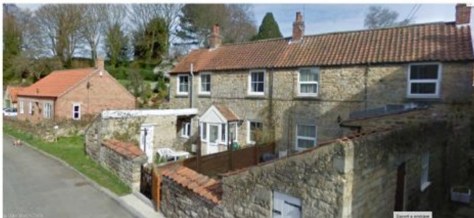
VIEW OF COTTAGES ON MANOR VALE LANE
