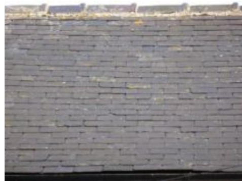
Natural slate roof
