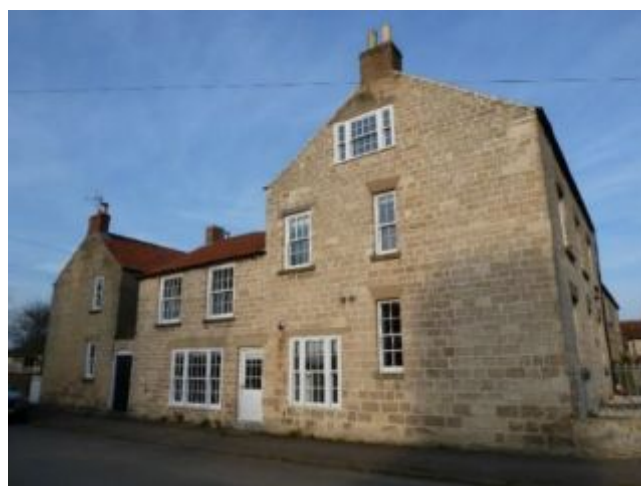
Lime pointing at Prospect House
